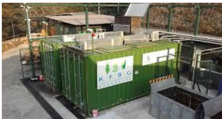
FIGUR 11 EARTH SYSTEMS BOKOLPANNA MPP20 FOTO: EARTH SYSTEMS
